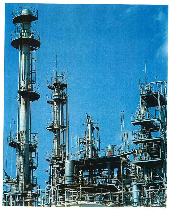
Toyo Soda is the biggest manufacturer of ethyleneamines in Japan. Above shown is the Shin-nanyo Plant which has a production capacity of 10,000 tonne/year. Toyo Soda developed its own process for producing ethyleneamines from ethylene dichloride in 1967. The process technology was licensed to Delamine BV in the Netherlands; the plant went on stream there in August, 1978 has a capacity of 15,000 tonne/year.
