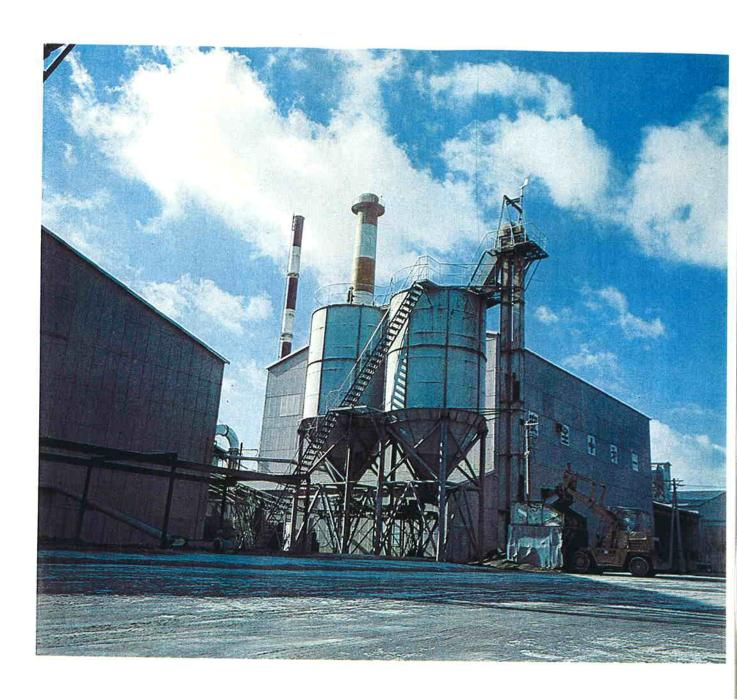
Ishinomaki Plant, built in a 74,000 m<sup>2</sup> site at Ishinomaki, Miyagi, in 1968, is capable of producing 50,000 tons per year of fused magnesium phosphate by the open-hearth furnace process.
